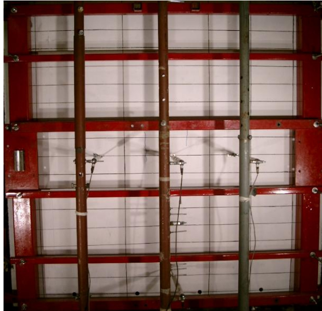
Figure 6.32: Condition of Wall 2 after test 2
