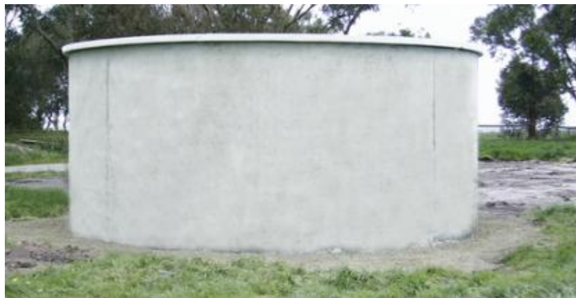
Figure 1.1: A circular concrete reservoir (AMCO Water 2014)
