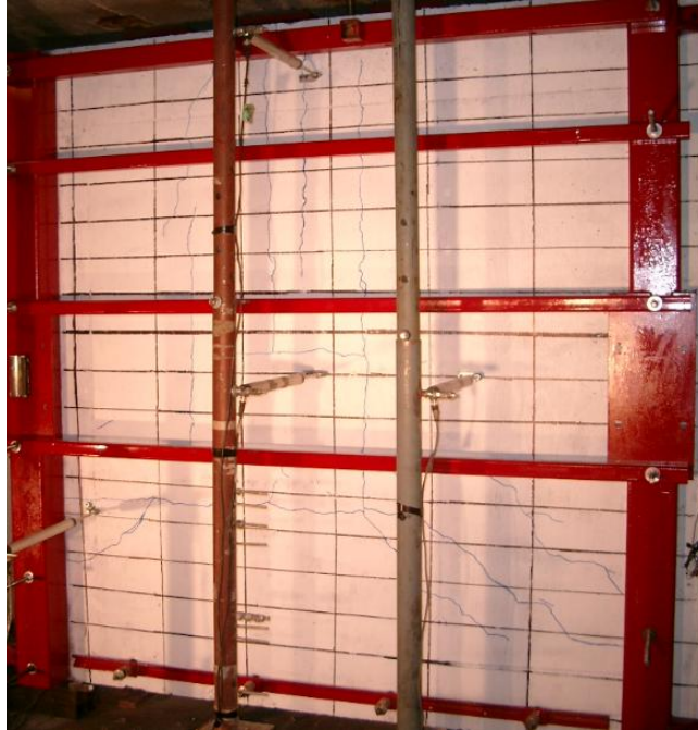
Figure 6.12: Condition of Wall 1 after test 3
