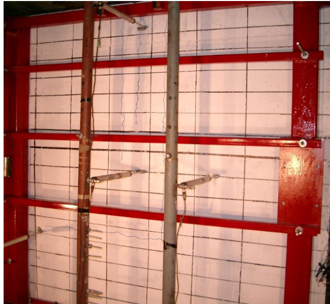
Figure 6.8: Condition of Wall 1 after test 2
