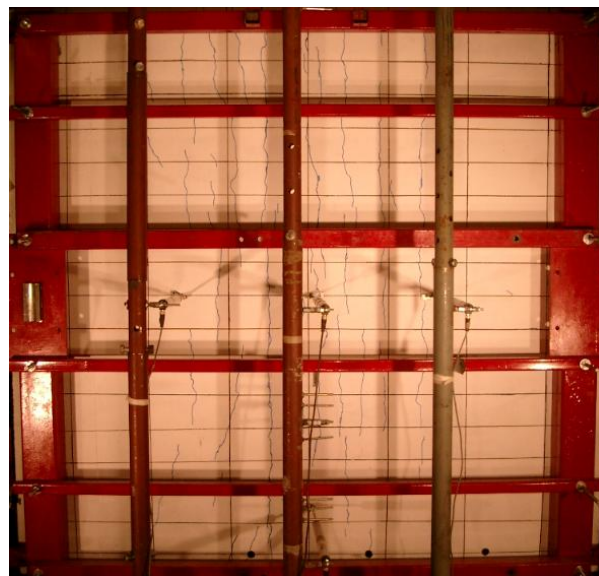
Figure 6.44: Condition of Wall 2 after test 5
