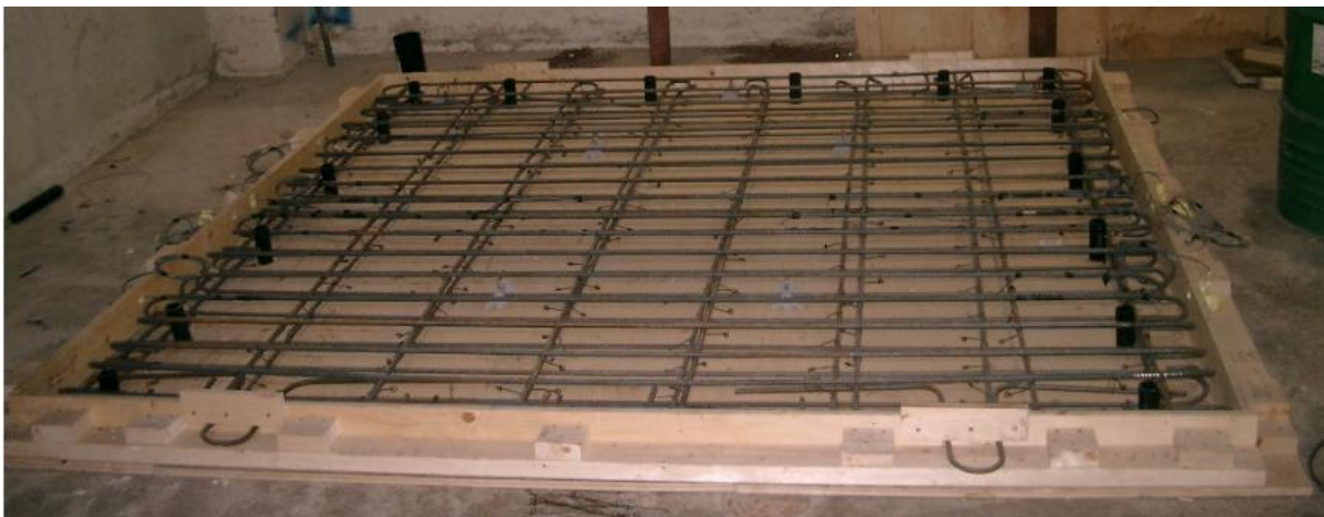
Figure 5.6: Wall specimen with reinforcement cage prior to casting
