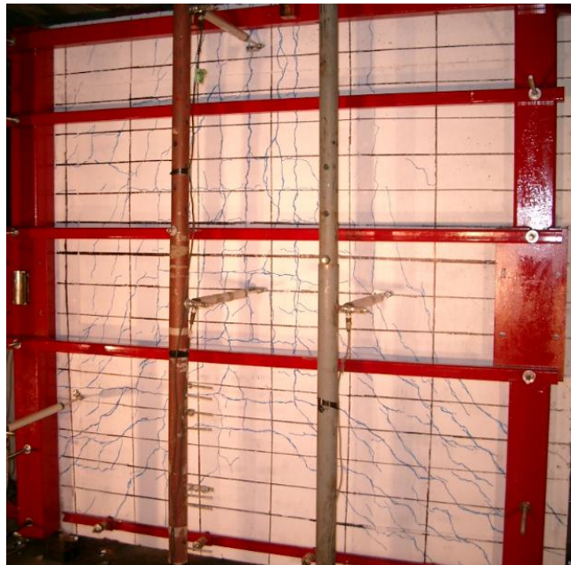
Figure 6.24: Condition of Wall 1 after test 6
