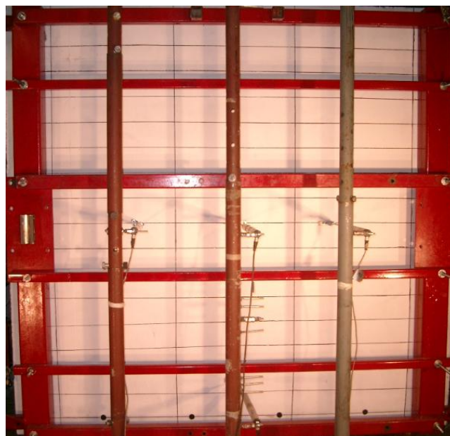
Figure 6.28: Condition of Wall 2 after test 1
