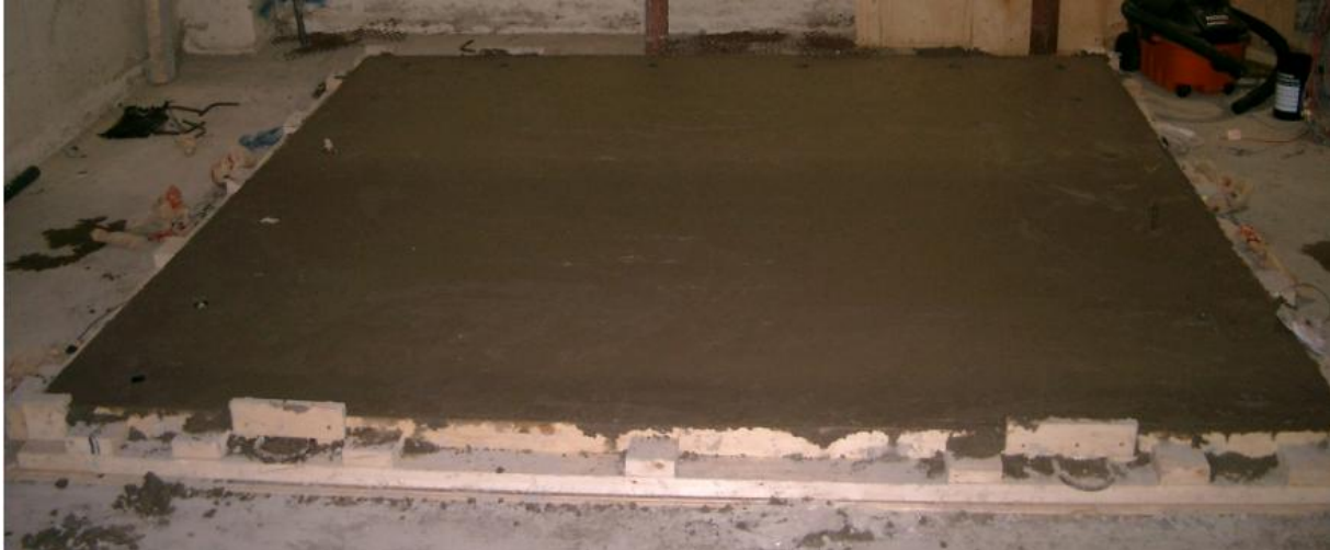
Figure 5.7: Reinforced concrete wall during casting
