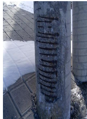
(b) Underpass in Bells Corners, Ottawa
