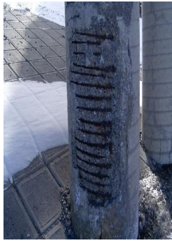
(b) Underpass in Bells Corners, Ottawa
