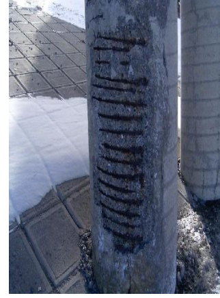
(b) Underpass in Bells Corners, Ottawa
