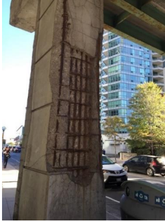
(a) Toronto Gardiner Expressway
