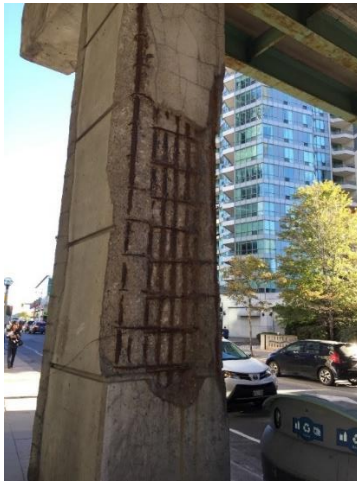
(a) Toronto Gardiner Expressway
