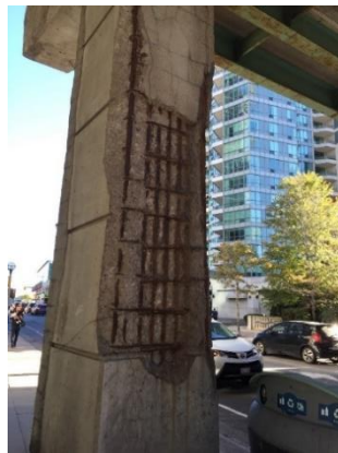
(a) Toronto Gardiner Expressway
