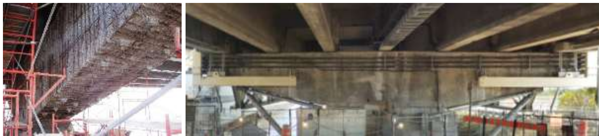
Figure 4-2 Images depicting the pier cap following removal of the surface concrete in 2004 (left) and in 2018 after addition of external longitudinal reinforcement and the modular truss system in 2018 (right). (reproduced from JCCBI (left), Map data ©2022 Google (right))
