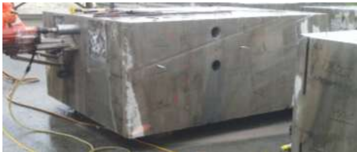
Figure 3-6 Image depicting core extraction from a pier cap segment at the Montreal storage site
