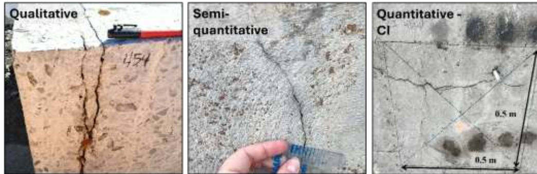
Figure 3-4 Images depicting qualitative, semi-quantitative and quantitative visual inspection
