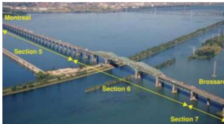
Figure 2-1 Annotated image identifying key sections of the Champlain Bridge (reproduced from [2])
