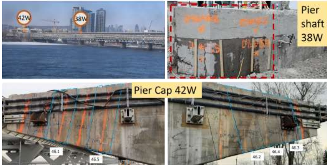
Figure 3-2 Annotated images depicting the concrete members under study and their location in the Champlain Bridge
