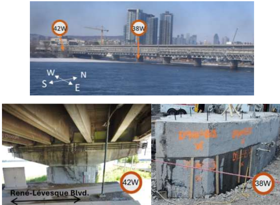
Figure 4-1 Annotated images identifying the location of the pier cap (42W) and pier shaft (38W). (Image sources: top and bottom right images courtesy of JCCBI, bottom left image: Map data ©2022 Google)
