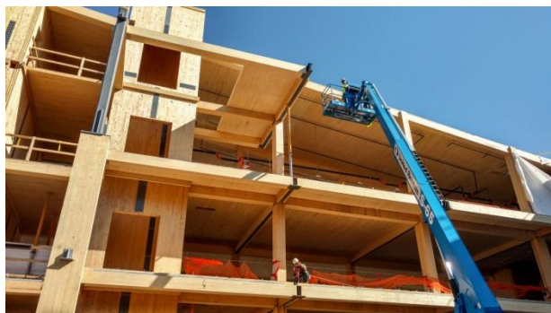
Figure 1.6: University of Massachusetts Design Building, Amherst, Massachusetts (Nordic Structures, 2017)
