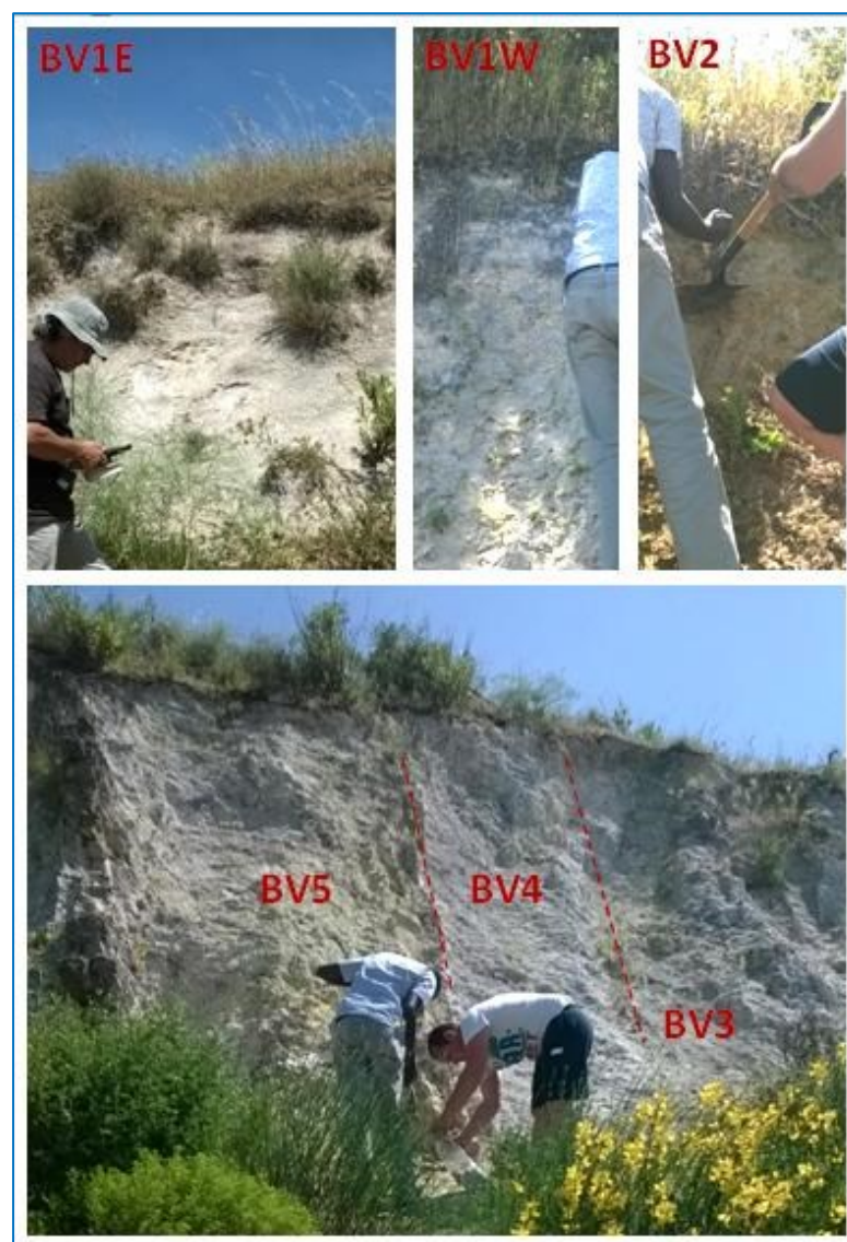
Figure 19. Detailed view on the Benavila sampling sites – BV5, BV4 and BV3 sampling sites significantly differ in color (BV3,BV5 – greenish; BV4 – grayish). The discontinuity in color correlates with a presence of a fault zone - photos by C. Costa, University of Aveiro, 2014.
