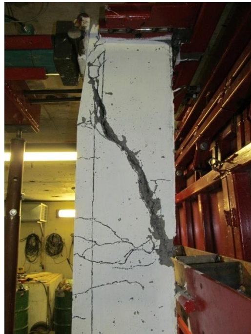
(b) Shear Failure of Blast 3
