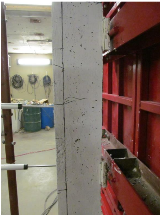
(a) Mid-Span Results of Blast 2
