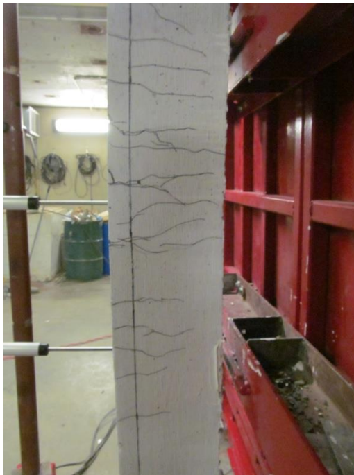
(a) Mid-Span Results of Blast 3
