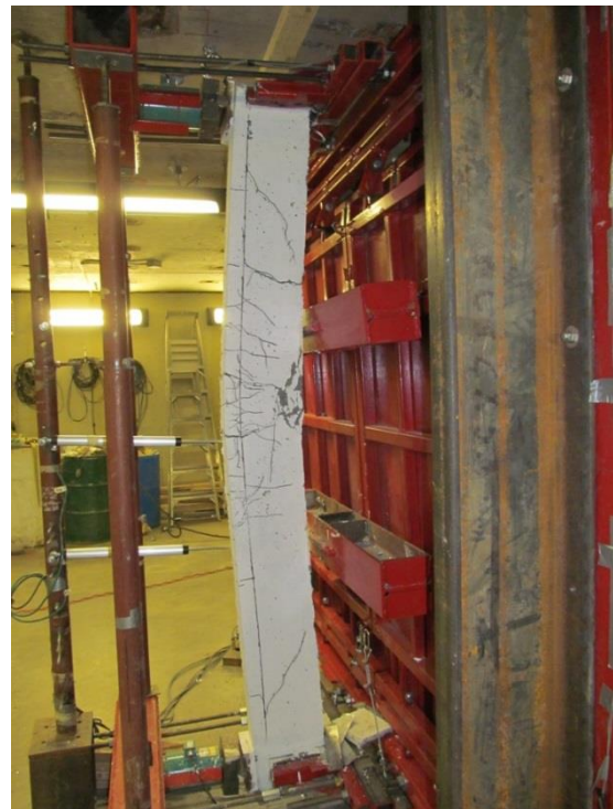
(b) SCC 0.75% BP flexural failure at Blast 4
