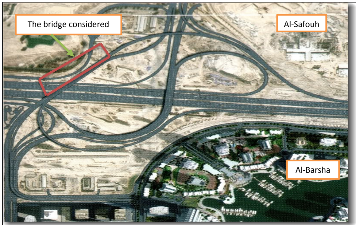
Figure 7.10: The bridge considered for the case study (areal photo for Sheik Zayed Road, Dubai-UAE, Google map).
