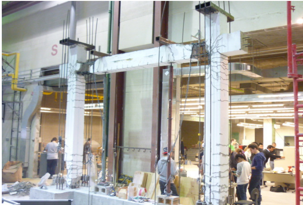
Figure 6.27: Bare control frame before placing repair formwork
