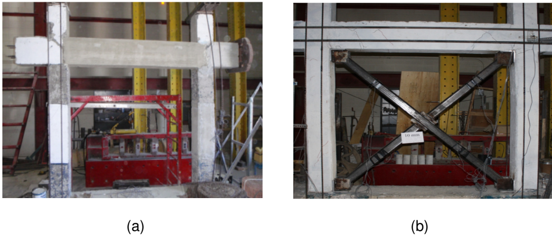
Figure 2.5: Seismically deficient frames prior to testing: a) repaired frame BR-3R; and b) repaired and retrofitted frame BL-3R (Caron 2010)
