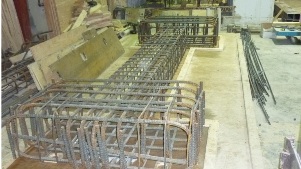
Figure 6.4: Construction of foundation reinforcement cage
