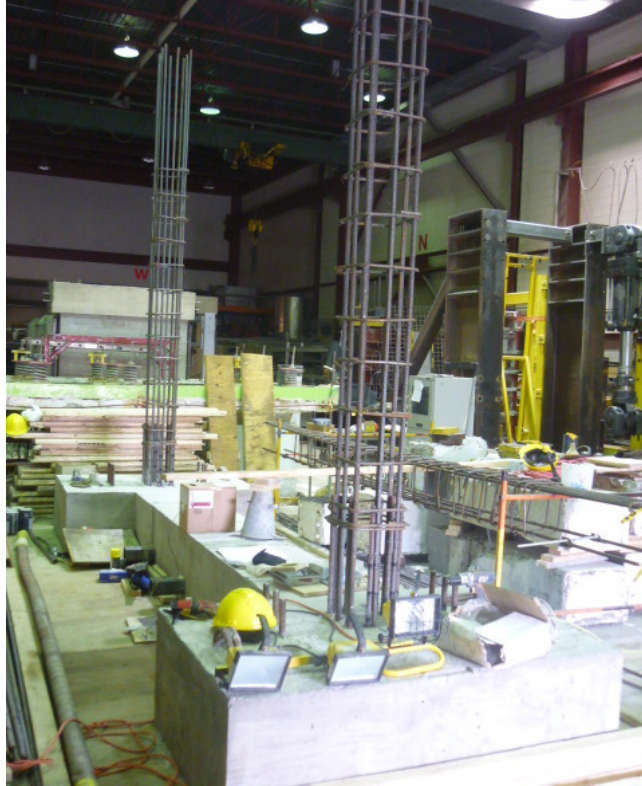
Figure 6.8: Placement of column longitudinal and transverse tie reinforcements
