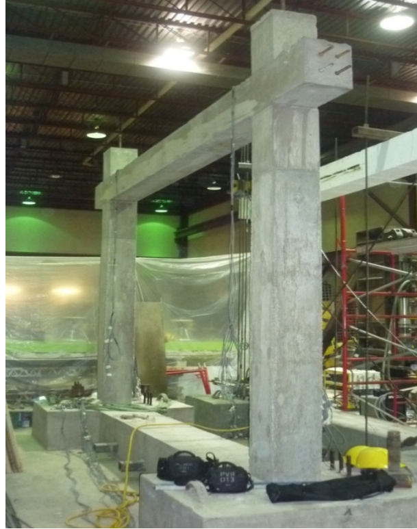
Figure 6.13: Frame specimen after concrete casting
