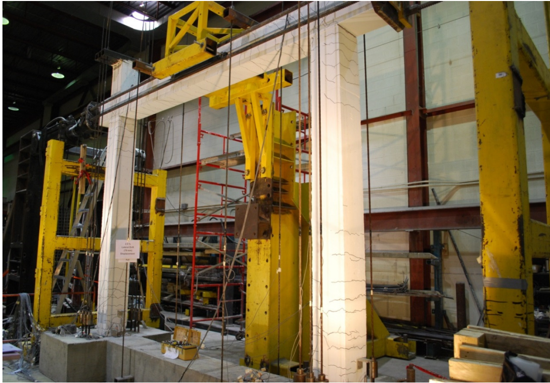
Figure 7.11: Cracking pattern at 2.5% lateral drift for Frame BCF
