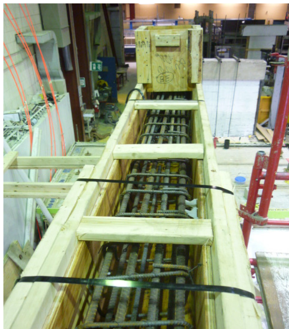
Figure 6.12: Placement of frame beam reinforcement
