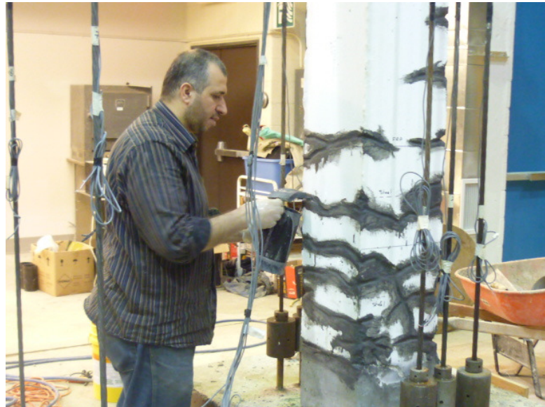
Figure 6.32: Application of bonding agent (SikaTop Armatec 110 EpoCem) prior to patching with mortar
