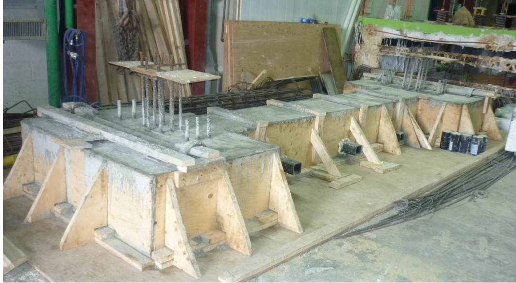
Figure 6.6: Concrete casting of the fame foundation
