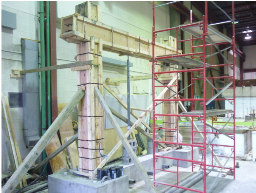
Figure 6.11: Construction of formwork prior to placement of beam reinforcement and concrete casting
