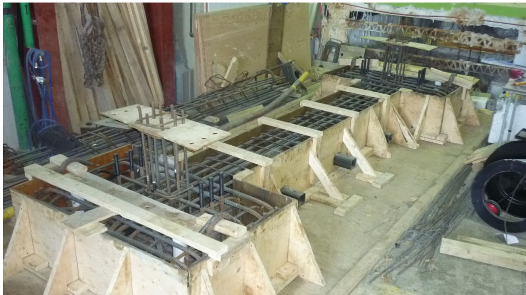
Figure 6.5: Foundation formwork and reinforcement cage with embedded column starter bars
