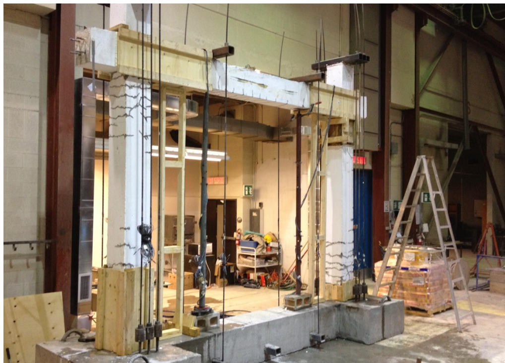
Figure 6.28: Formwork before casting the new self-compacting concrete (Sikacrete-08 SCC)
