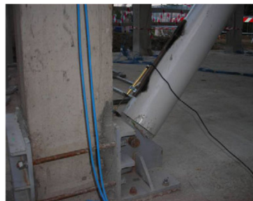
BRB connection to column
