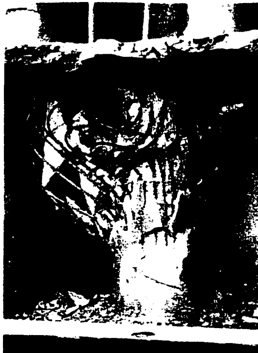
Figure 1.4 Column failure of Interstate 10 highway bridge undercrossing at Lacienea and Venice during the 1994 Northridge Earthquake. (Saatcioglu, 1994:)
