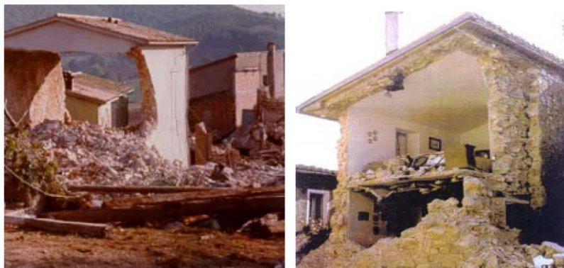
Figure 1-1. Out-of-plane failures of load-bearing walls, Umbria, Italy, 1997 (Babaeidarabad, 2013)
