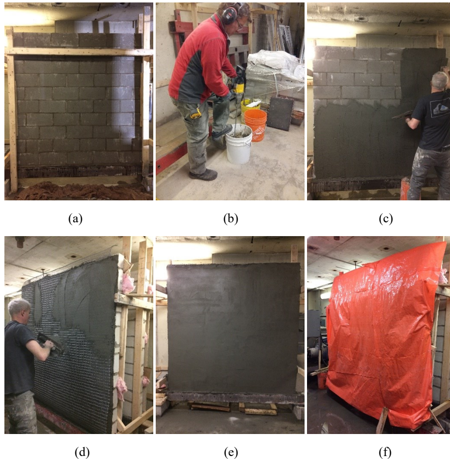
Figure 3-7. FRCM application: (a) Surface Preparation, (b) Mortar mixing, (c) Base mortar (1/2''), (d) Additional mortar (1/4''), (e) Final mortar (1/2''), (f) Water curing with burlap and plastic tarp
