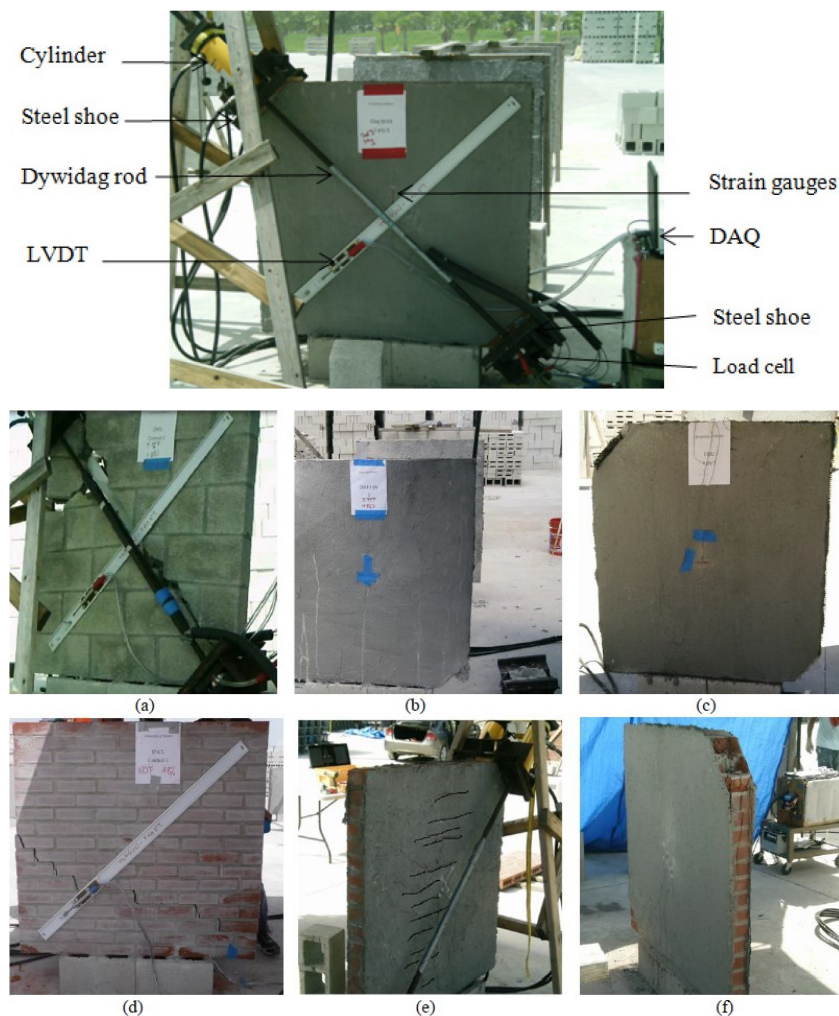
Figure 2– Failure mode of wall specimens: CMU-Control (a); CMU-1ply (b); CMU-4ply (c); CL-Control (d); CL-1ply (e); and CL-4ply (f)
