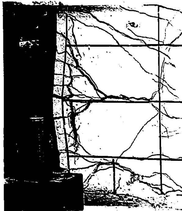
Figure 3.7: Buckling of exterior flexural bars
