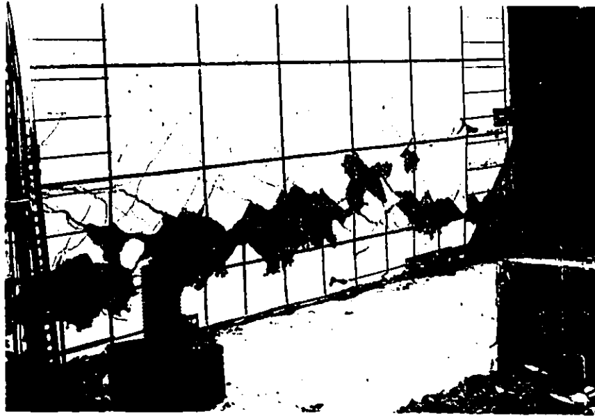
Figure 3.37: Wall 6 at the end of the test
