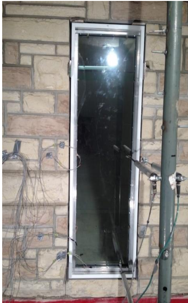
Figure B.34: Photograph of ST5 after testing
