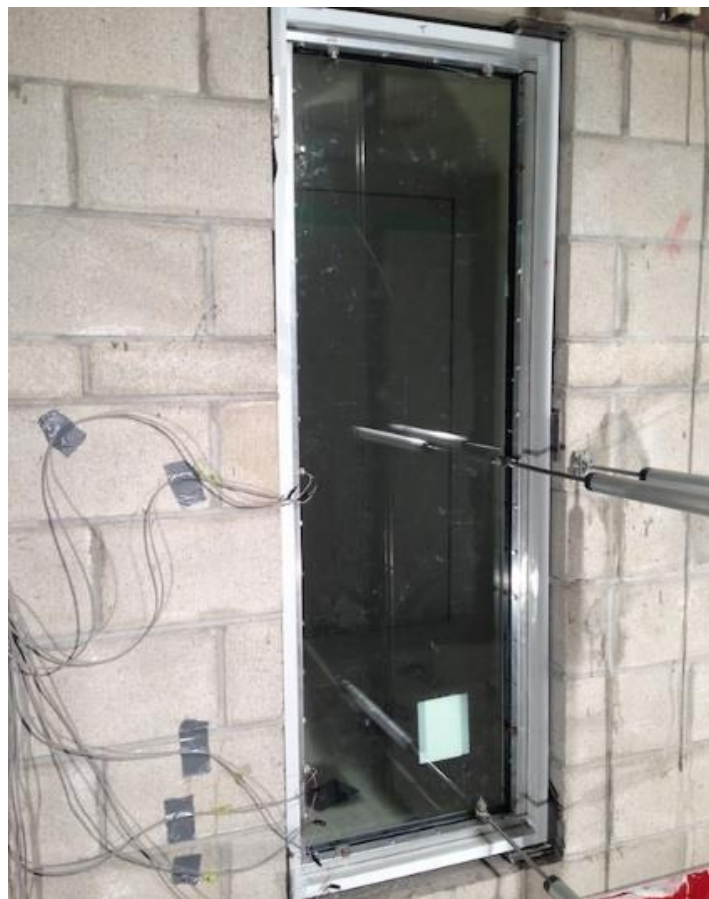
Figure B.20: Photograph of B9 after testing
