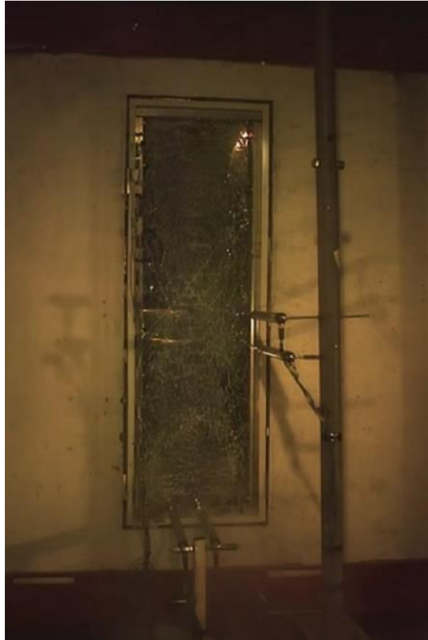
Figure A.12: Photographs of C6 after testing
