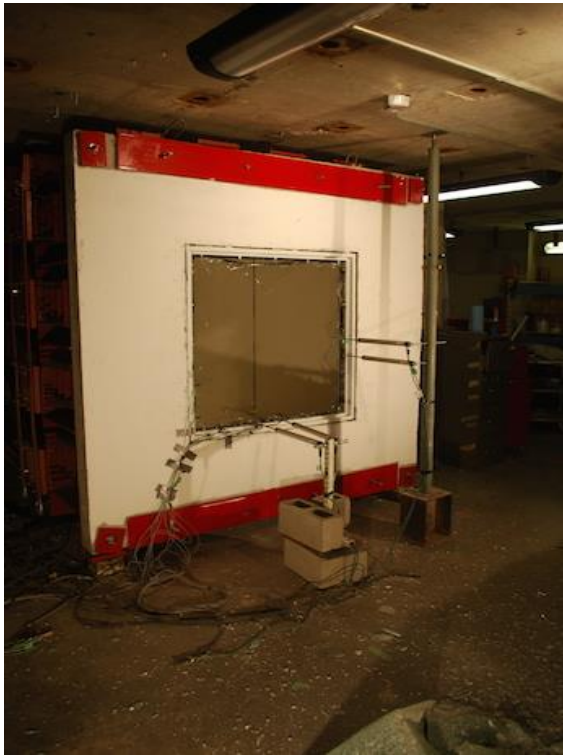
(c) Window after Test C4
