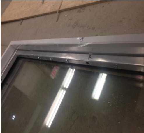
(b) Mechanical glazing
