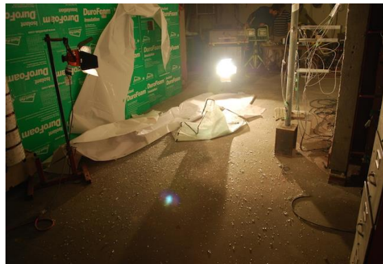
(d) Damaged witness panel and glazed pane on the floor after Test C2
