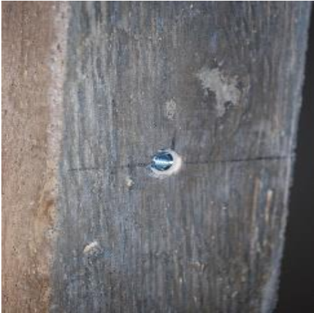
Figure 3.4: Drop-in anchors
