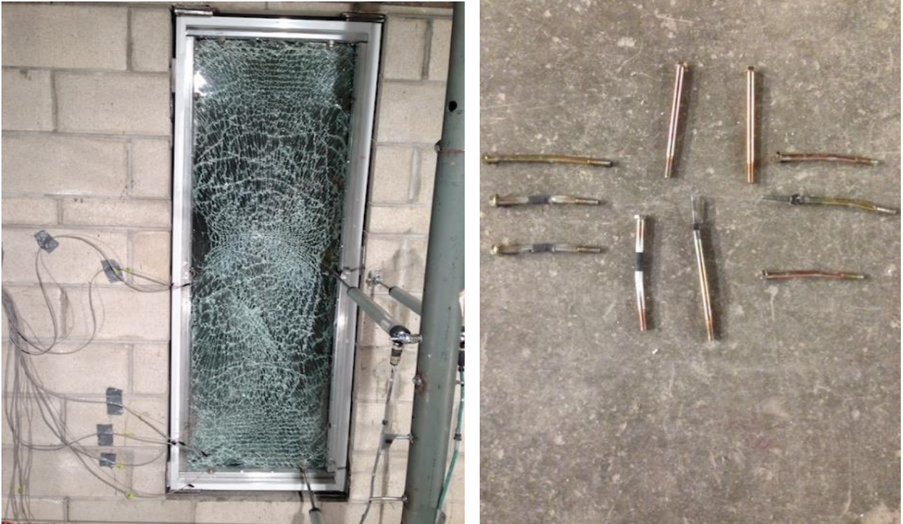
Figure B.22: Photographs of window and anchors after Test B10
