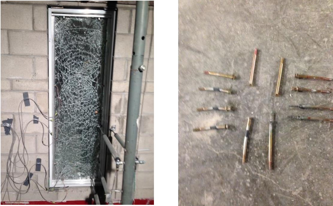
Figure B.18: Photograph of window after Test B8
