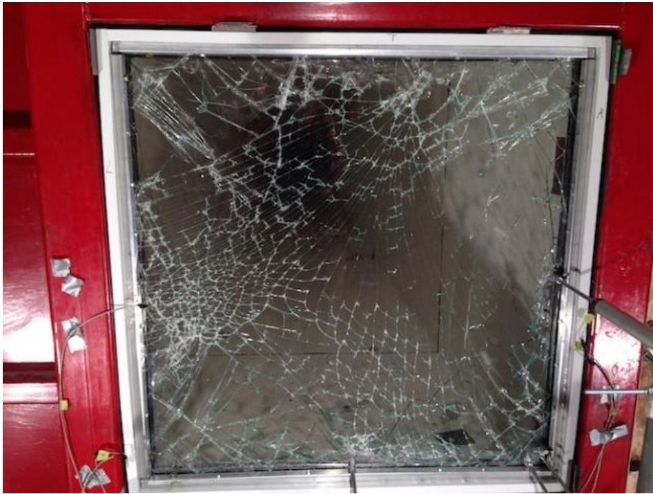
Figure A.55: Photograph of S11 after testing
