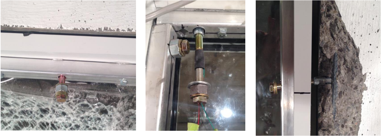
Figure 4.5: Anchorage pull-out during tests
