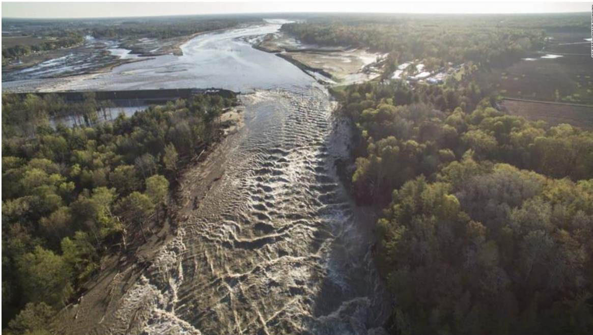
Figure 1.1. Edenville Dam failure. Photo editing by Sarah Tilotta, 20 May 2020
