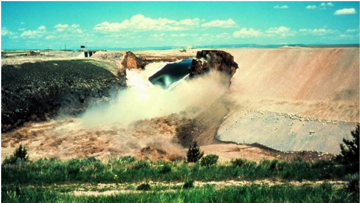
Figure 3.1. Teton Dam Failure; northwest view toward the breach. Photo by Mrs. Eunice Olson, 5 June 1976.
