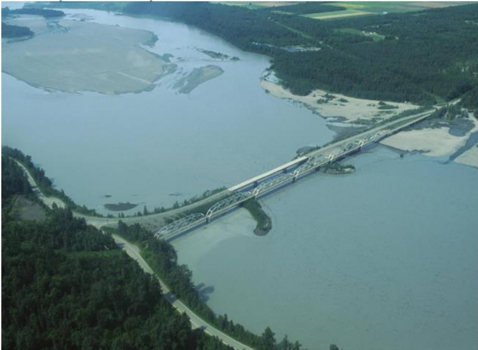
Figure 14: A bridge built across the Knik River, Alaska. Guidebanks result in a channel constriction thus the river is subject to both local and constriction scour (courtesy of Jeff Conway, United States Geological Survey)
