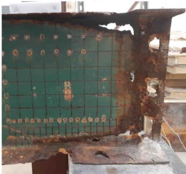
Figure 2- 4: Bridge B specimen 5 – thickness (Tzortzinis, 2021)
