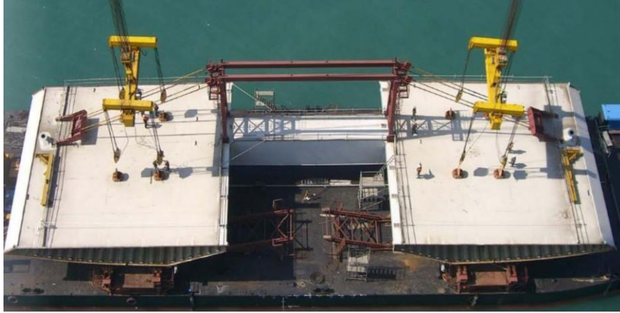
Figure 3- 1: One segment of Stonecutters Bridge Deck (Sabri, 2013)
