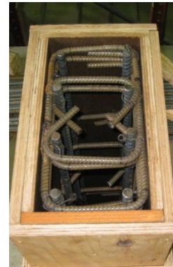
(e) Specimens “Without Cover” in Formwork
