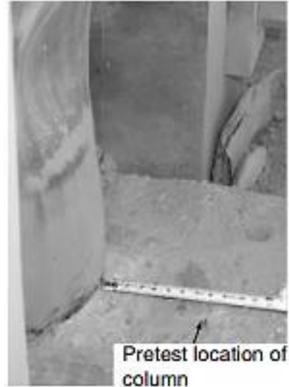
(b) Direct Shear Failure
