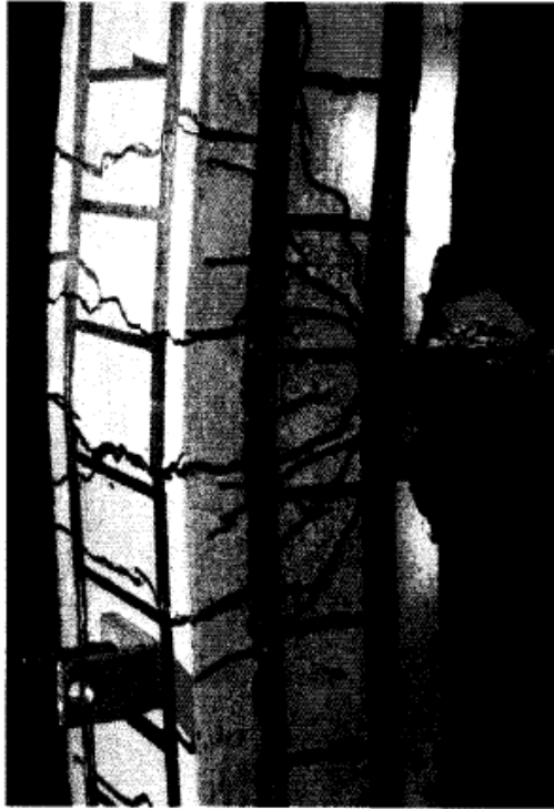
Figure 2-18: Flexural Cracks at the Mid-Span of the Column (Lloyd 2010)
