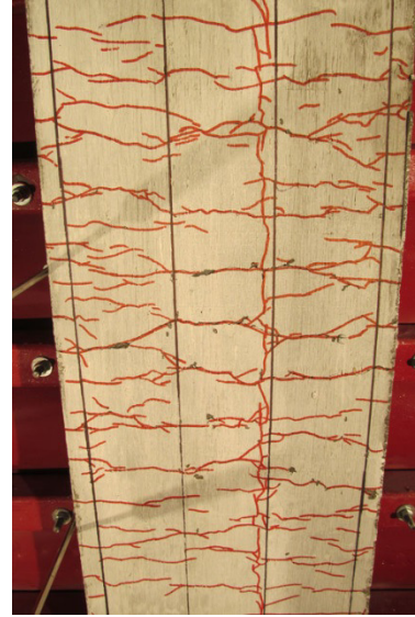
b) SCC-1.2%ZP-#3HS-100 Minimal cracking after Blast 4
