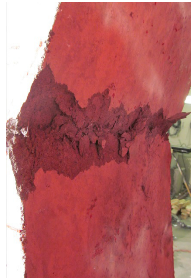
h) Concrete crushing at Blast 5
