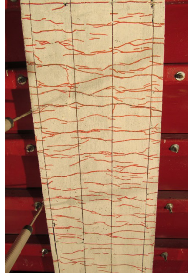
c) CRC-2%A-#3HS-100 Tensile cracking after Blast 5
