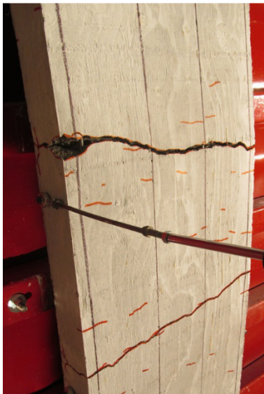
d) Mid-span cracking at Blast 2
