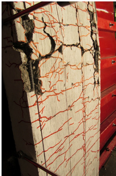
g) Mid-span cracking at Blast 5
