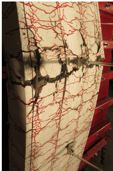
e) SCC-1.2%ZP-#3NS-100 Improved crack control at Blast 5
