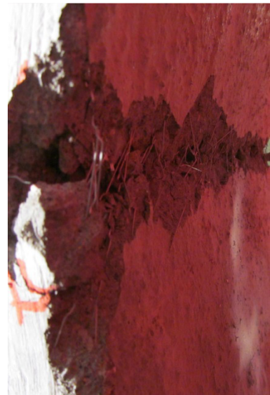
g) Concrete crushing at Blast 4
