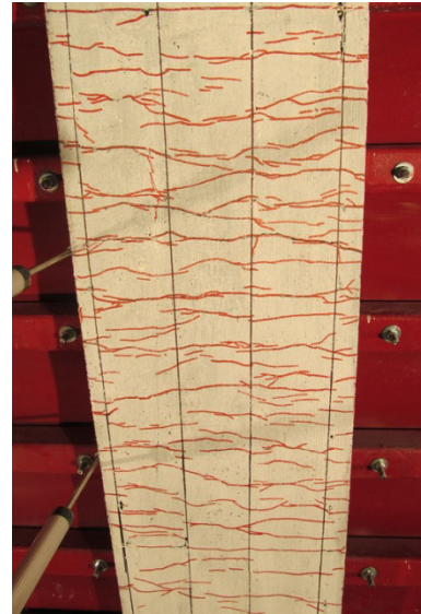
c) CRC-2%A-#3HS-100 Tensile cracking at Blast 5
