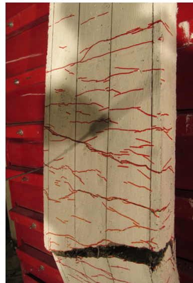
f) CRC-2%A-#3NS-100 Bar rupture at Blast 5
