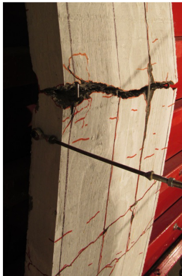
e) Mid-span cracking at Blast 3
