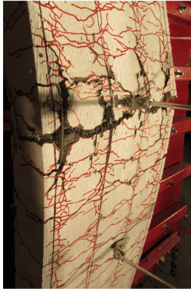
g) Mid-span cracking at Blast 5
