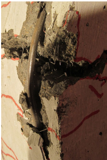
d) SCC-1.2%ZP-6.3NS-80 Bar slippage at Blast 4
