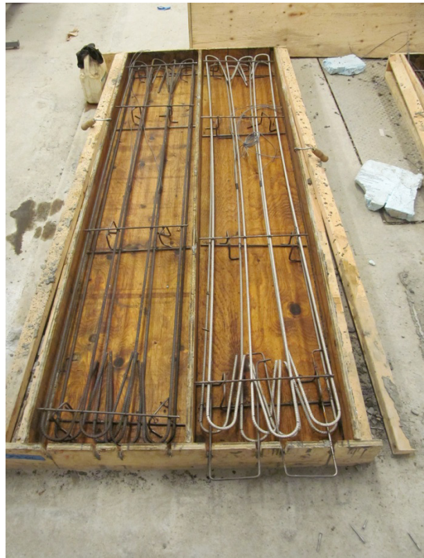
b) High strength / Stainless steel reinforcement
