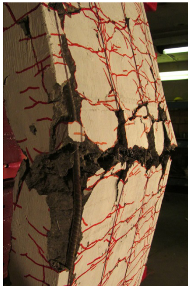
g) Mid-span cracking at Blast 5
