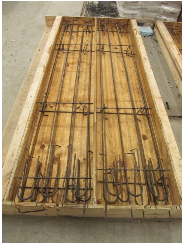
a) Regular steel reinforcement
