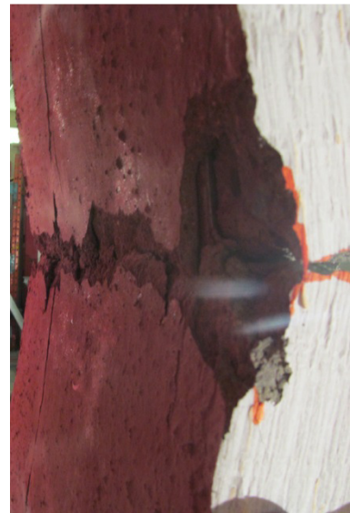
f) Mid-span crushing at Blast 3
