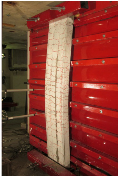
g) Vertical cracking at Blast 5
