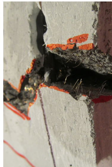
e) CRC-2%B-6.3NS-80 Bar rupture at Blast 4
