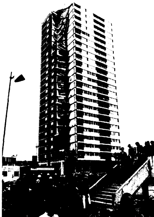
Figure 1.2 Partial progressive collapse of the Ronan Point Building in London, England (from Shankar 2004).
