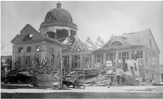
Figure 1.1: Damaged exposition building in Halifax, NS, after the 1917 explosion (George Grantham Bain Collection 2021)
