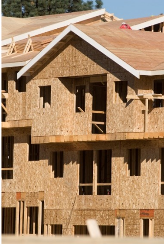
Figure 2.1: Light frame construction (naturallywood.com 2021)
