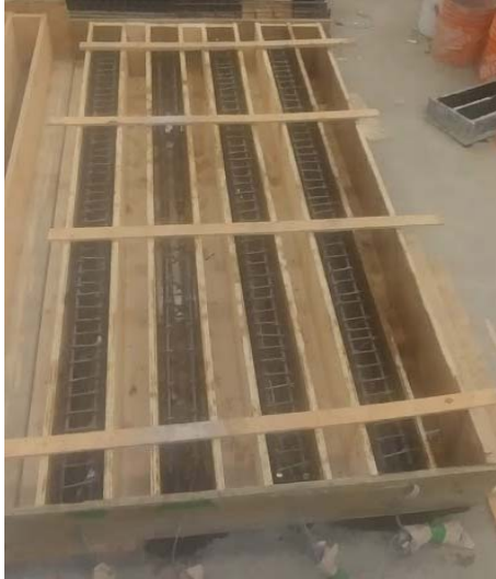
(a) Beams in formwork before casting
