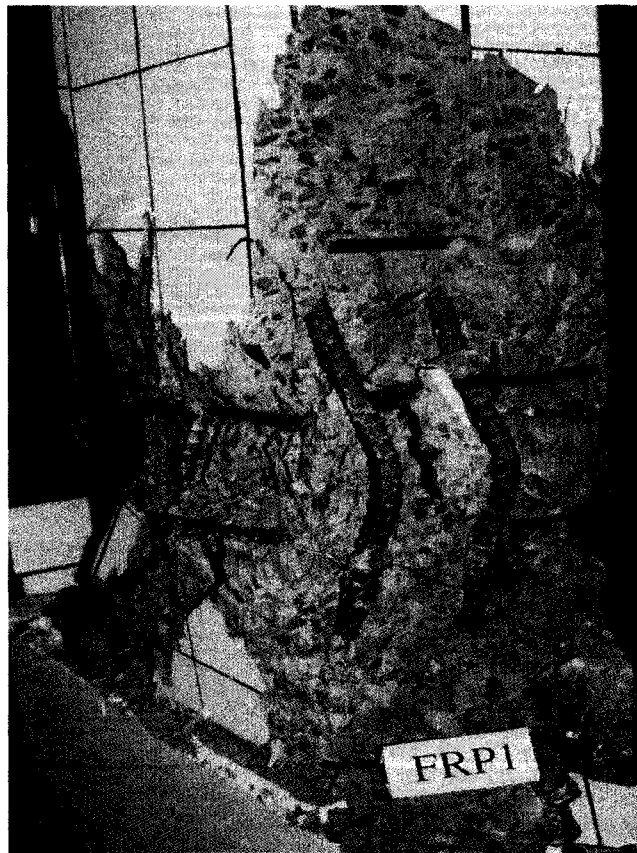
b) Steel bar buckling in compression
