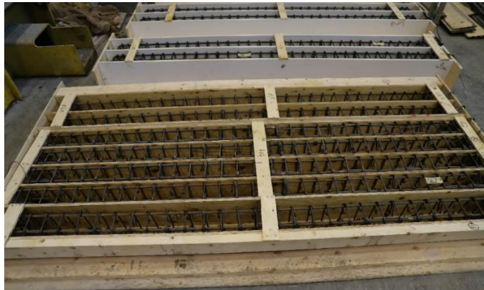
Figure 3 - 18 Formworks and steel gauges in series 2
