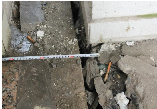
(b) Separation Gap around the Superstructure
