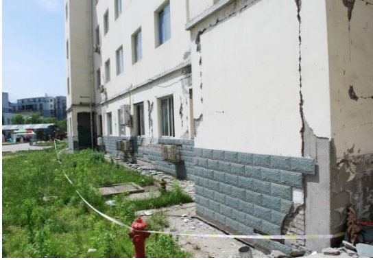
(a) Outside of the Building
