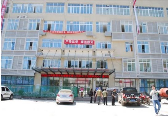
(a) Outside of the Building
