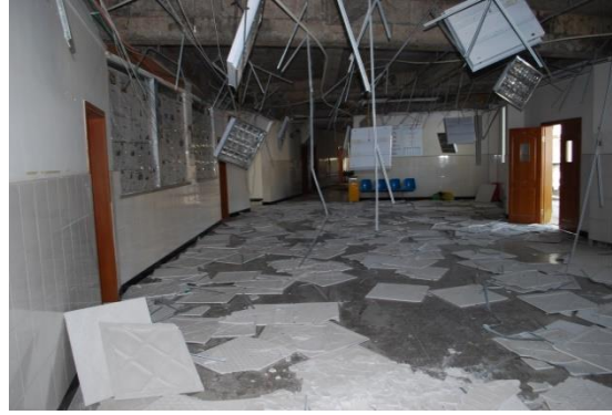
(b) Inside of the Building
