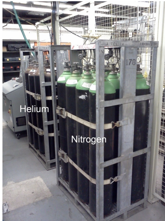
Figure 4.11 : Helium and nitrogen bottles packs
