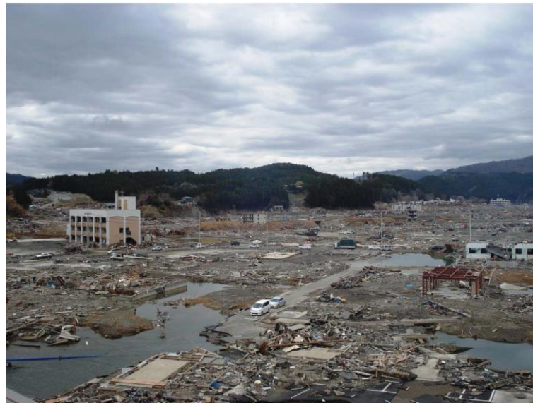
Figure 1.3: Extensive devastation of inland buildings during 2011 Tohoku Tsunami in Onagawa city, [Courtesy of Dr. I. Nistor].
