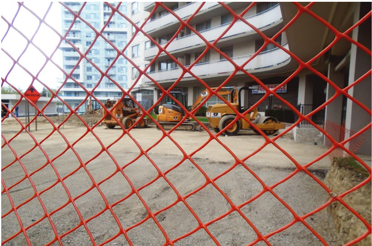
Figure 1 Construction site outside apartment building. Scarborough.
