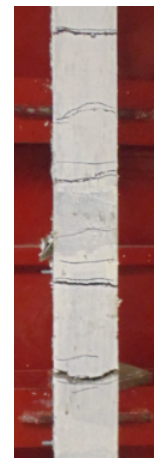
i) Mid-span concrete crushing/concrete splitting Tension face (Blast 7)
