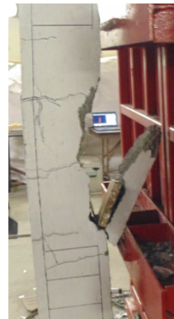
f) Mid-span concrete crushing (left side) (Blast 3)
