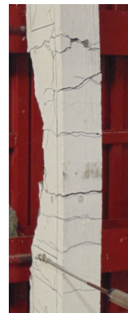
g) Mid-span cracking (East face) (Blast 4)
