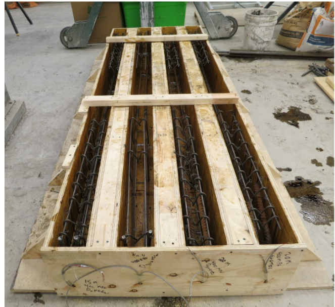
b) Formwork and Steel Cages
