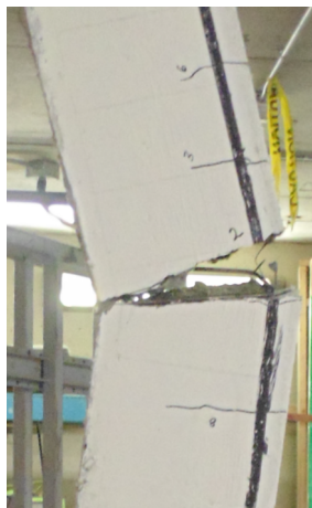
e) Mid-span cracking left side (Blast 4)
