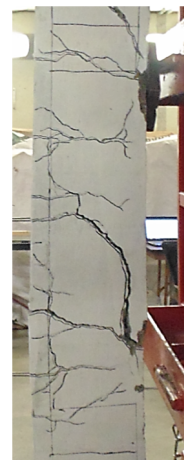
f) Mid-span cracking (north face) (Blast 3)
