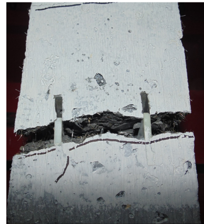
f) Mid-span fiber pullout (East face) (Blast 4)
