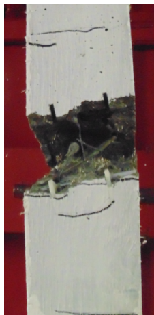
f) Mid-span cracking (Blast 4)
