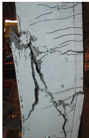
h) Mid-span concrete crushing/concrete splitting (Blast 7)
