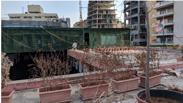
Figure 14 Parched ornamental plants on the roof of the school.
