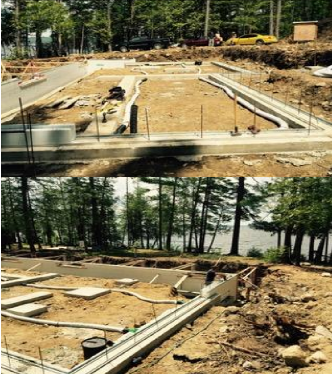
c. Placing of sub-slab perforated pipes during construction
