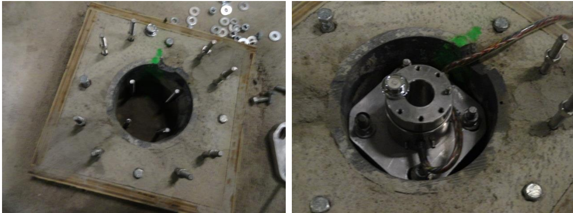
Figure 3.16: Left: Concrete pad with anchor bolts; Right: Force dynamometer levelled and secured in well
