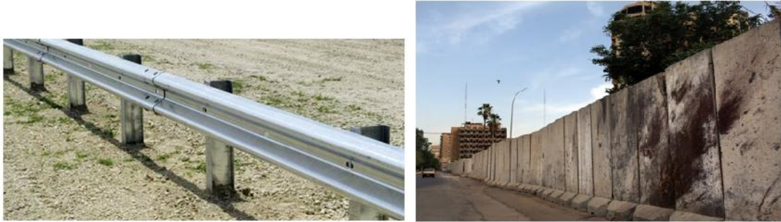
Figure 2-24: Examples of sacrificial barriers: guardrail (left) and blast wall (right)
