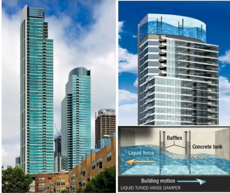
Fig. 1.1. Installation of a Tuned Liquid Damper (TLD) in Tall Buildings
