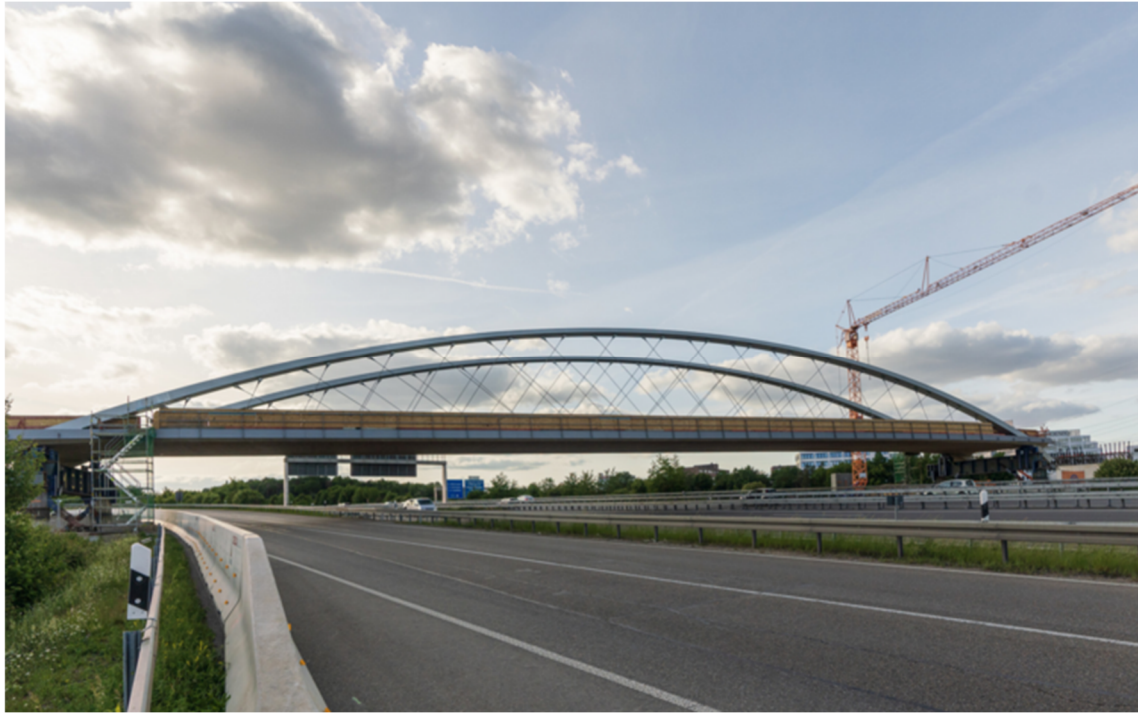
Figure 3 – Stuttgart Stadtbahn Bridge using Carbo-link CFRP Hangers [40]
