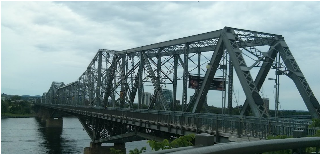
Figure 6 – Existing Alexandra Interprovincial Bridge
