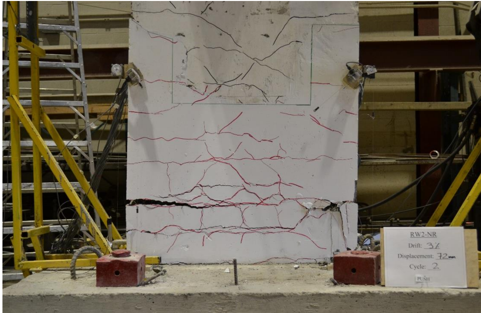
Figure A.2.9: Crack Pattern of Wall RW2-NR at 3% Drift (72 mm Displacement)
