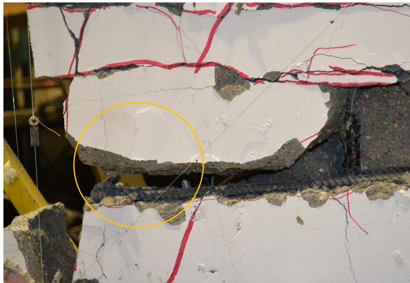
Figure 4.11: Rupture of Reinforcing Bars in Boundary Zone of RW1-SR
