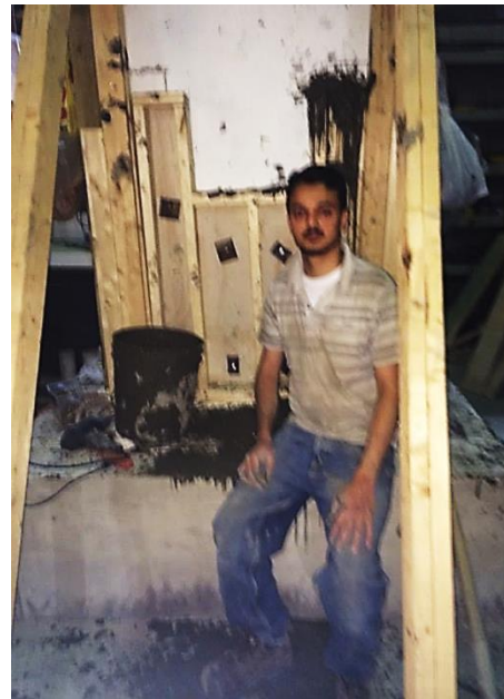
Figure 3.22: Casting of Concrete
