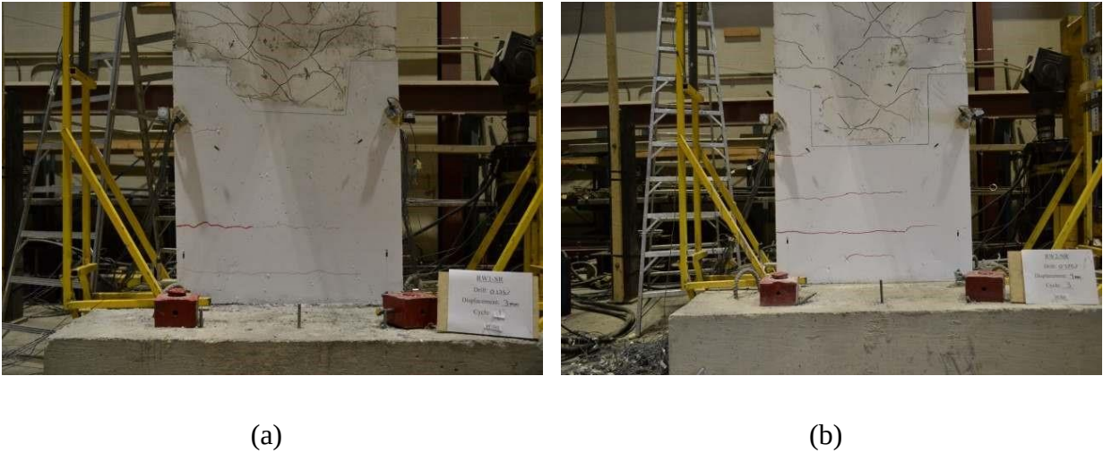
Figure 4.1: Initial Flexure Crack Pattern: (a) RW1-SR; and (b) RW2-NR
