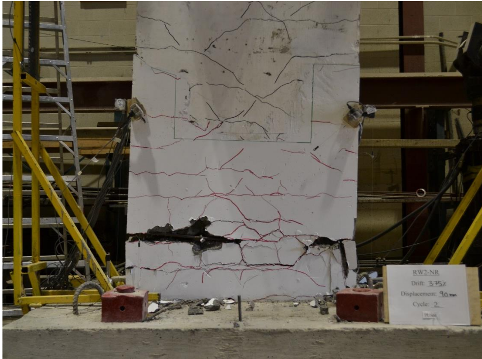
Figure A.2.11: Crack Pattern of Wall RW2-NR at 3.75% Drift (90 mm Displacement)
