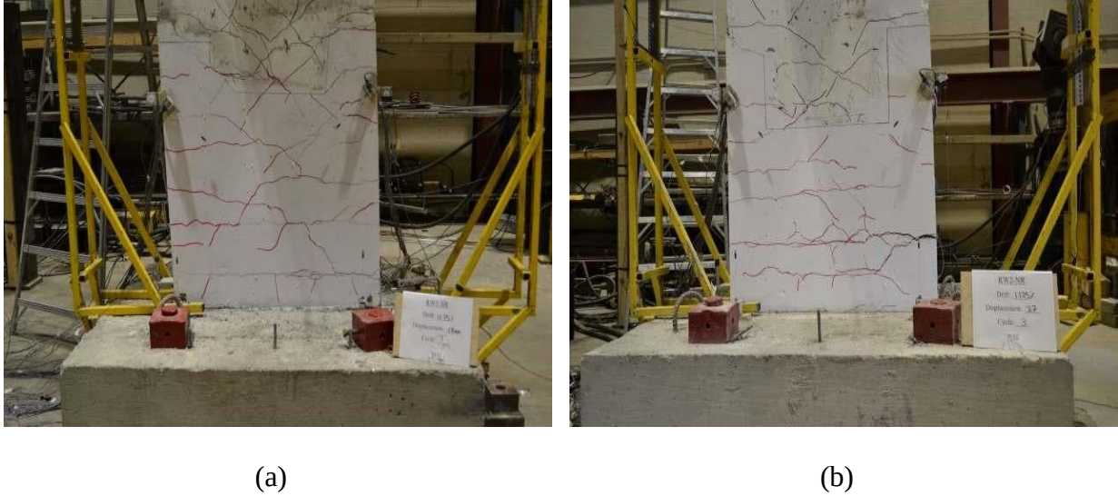
Figure 4.3: Post-Yield Crack Pattern at Drift Level of 1.12%: (a) RW1-SR; and (b) RW2-NR
