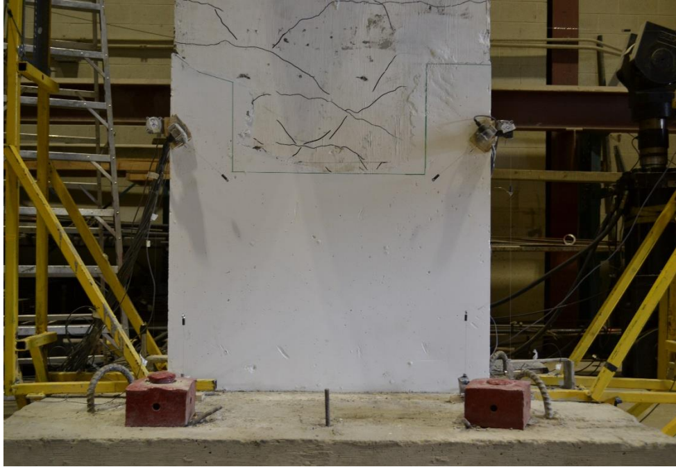
Figure A.2.1: State of Wall RW2-NR Before Testing
