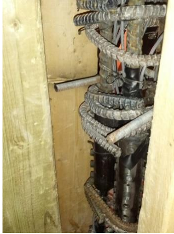
Figure 3.19: Additional Bars to Maintain Uniform Cover
