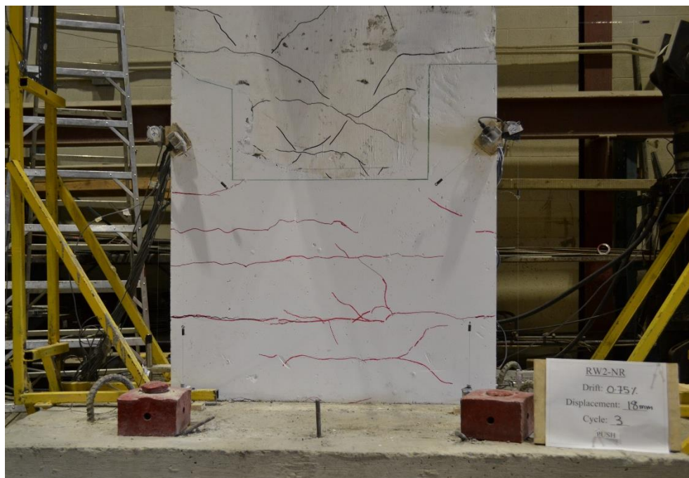
Figure A.2.3: Crack Pattern of Wall RW2-NR at 0.75% Drift (18 mm Displacement)
