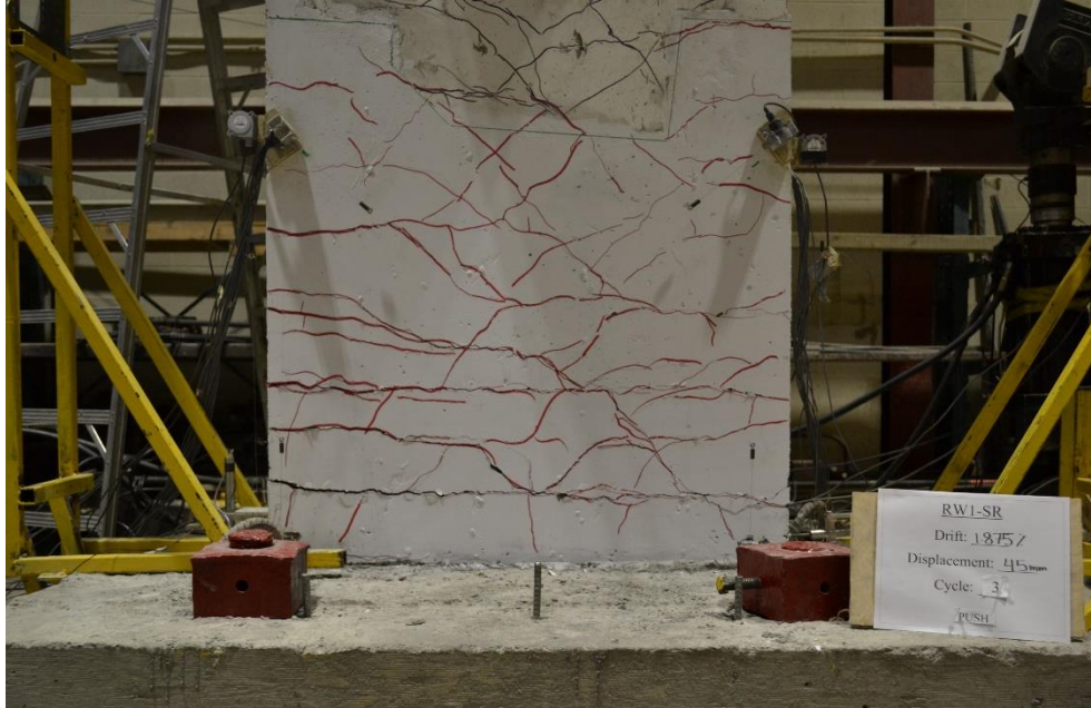
Figure A.1.8: Crack Pattern of Wall RW1-SR at 1.875% Drift (45 mm Displacement)
