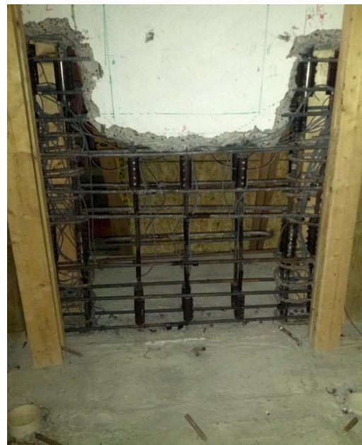
Figure 3.12: Reinforcement Layout in the Repaired Region of RW2-NR
