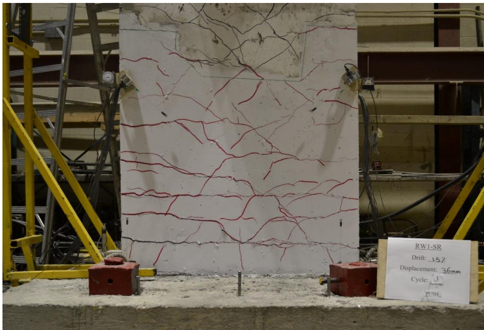
Figure A.1.7: Crack Pattern of Wall RW1-SR at 1.5% Drift (36 mm Displacement)
