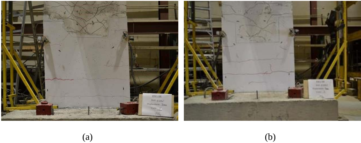
Figure 4.2: First Diagonal Crack: (a) RW1-SR; and (b) RW2-NR
