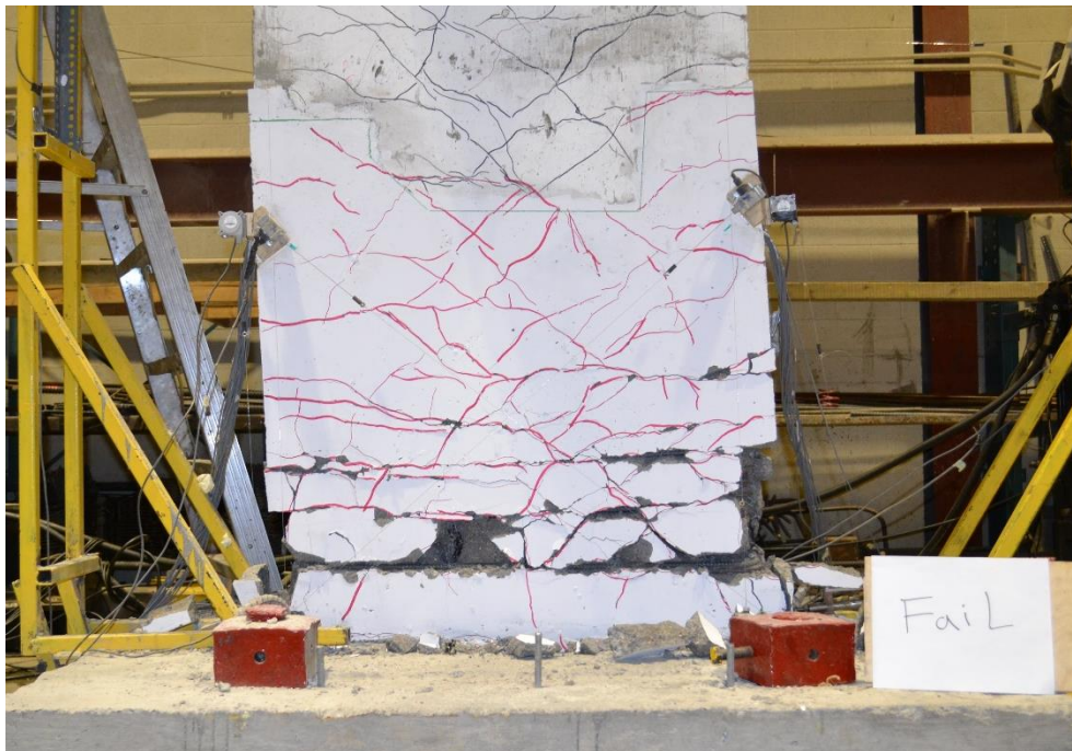
A.1.13: Crack Pattern of Wall RW1-SR at Failure
