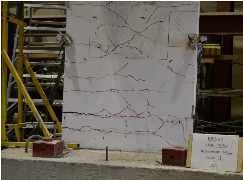
Figure A.2.6: Crack Pattern of Wall RW2-SR at 1.875% Drift (45 mm Displacement)
