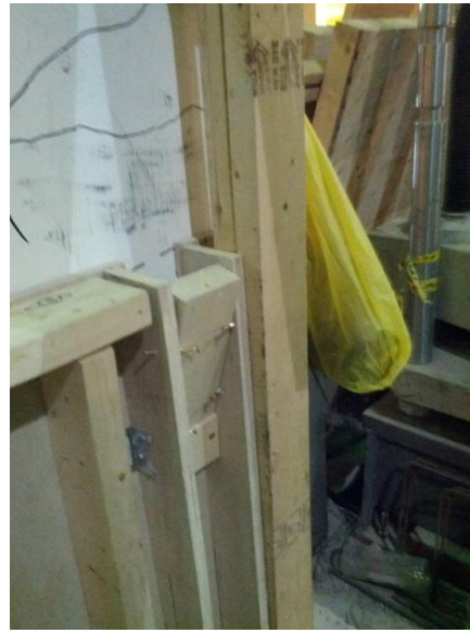
Figure 3.20: Form Work for Both Walls
