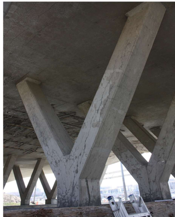
Figure 1-1. AAR damage extent on Robert-Bourassa Charest Overpass: a. Close up of the cracks on the side of the pier, b. Overview of the pier distress. Source: Sanchez et al. (2016).
