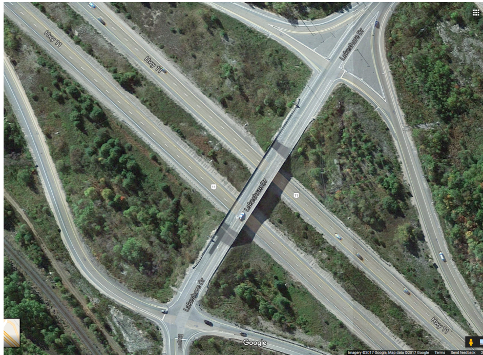
Figure 5.1 - Lakeshore Drive Bridge Aerial View (Google Earth™)
