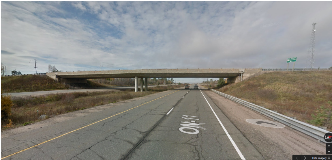
Figure 5.3 - Lakeshore Drive Bridge Side View with Highway ON-11 Underpass (Google Earth™)
