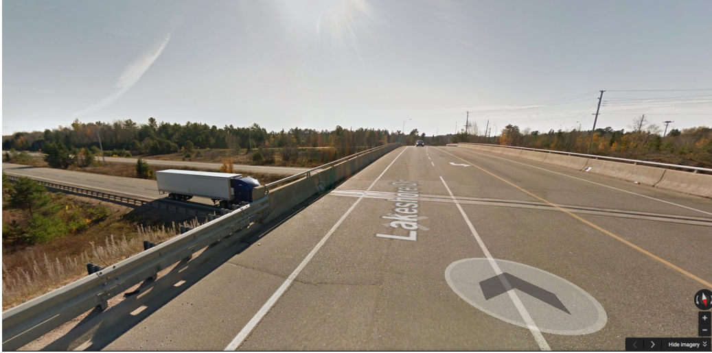
Figure 5.2 - Lakeshore Drive Bridge Deck View (Google Earth™)
