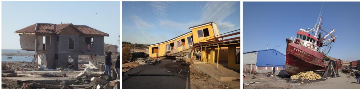
Figure 2.2 Experimental and numerical modelling of tsunami loading on structures by Nistor et al., (2011): Tsunami infrastructures damage due to the 2010 Chile earthquake and tsunami
