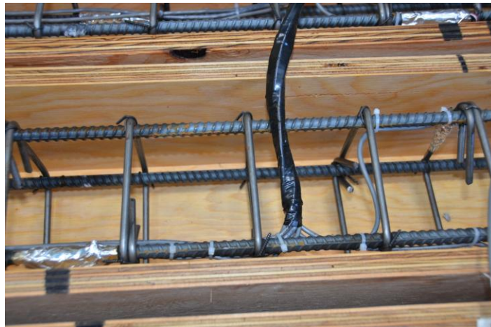
Figure 3. 18. Protected strain gauge assembly and taped wires to the rebar
