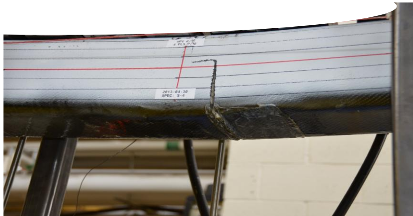
Figure 4.44. Damage to Column S4 at maximum load
