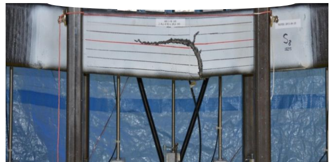
Figure 4.61. Damage on side face of Column S8 at maximum load
