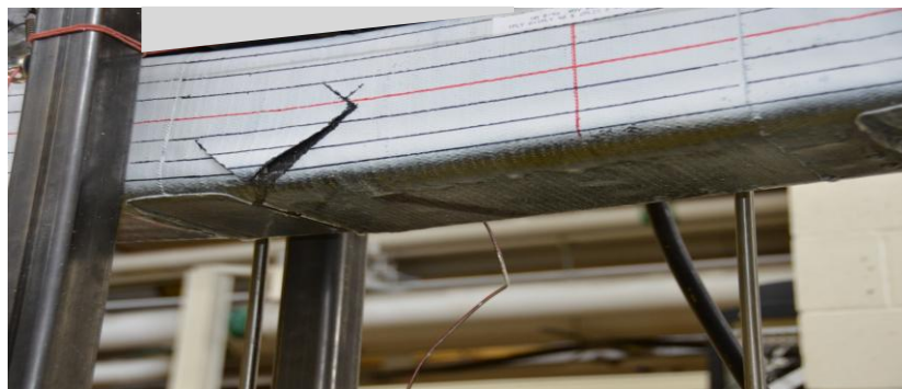
Figure 4.72. Damage to Column S3 at maximum load
