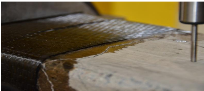
Figure 4.14. Damage to Column S6 near the roller support
