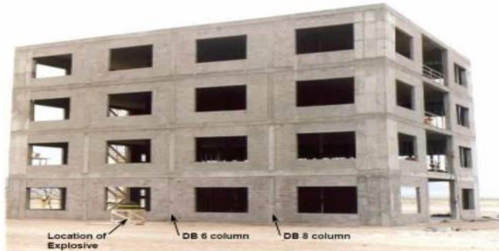
Figure 2.2: Test building for field testing and locations of DB 6 and DB 8 columns
