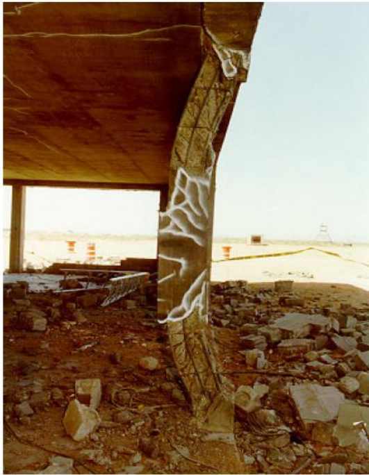
(a) Column from DB 6 test.
