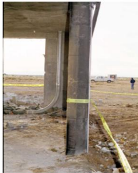
(b) Composite retrofitted column (DB 8)
