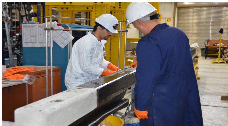
Figure 3. 20. FRP is impregnated in resin and the air is rolled out from the saturated fabric
