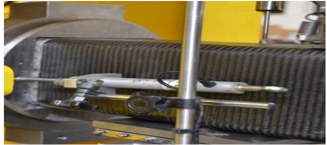
Figure 4.50. Damage to Column S7 near the roller support
