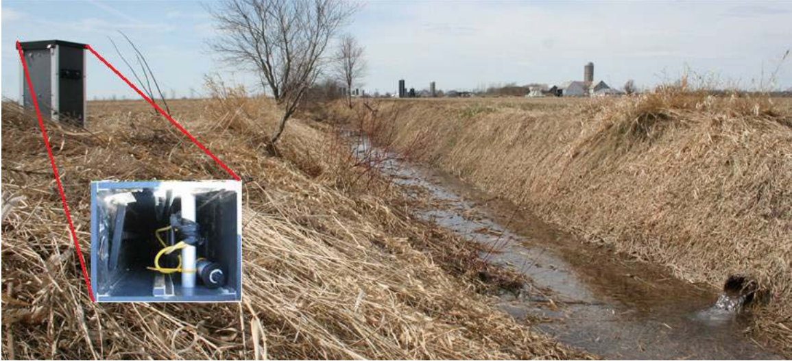
Figure 35 dam structure outlet of CTD
