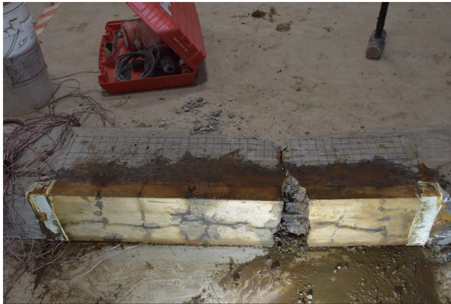
Figure B.21: Corrosion-induced damage in the cover of concrete – beam LS-2.1
