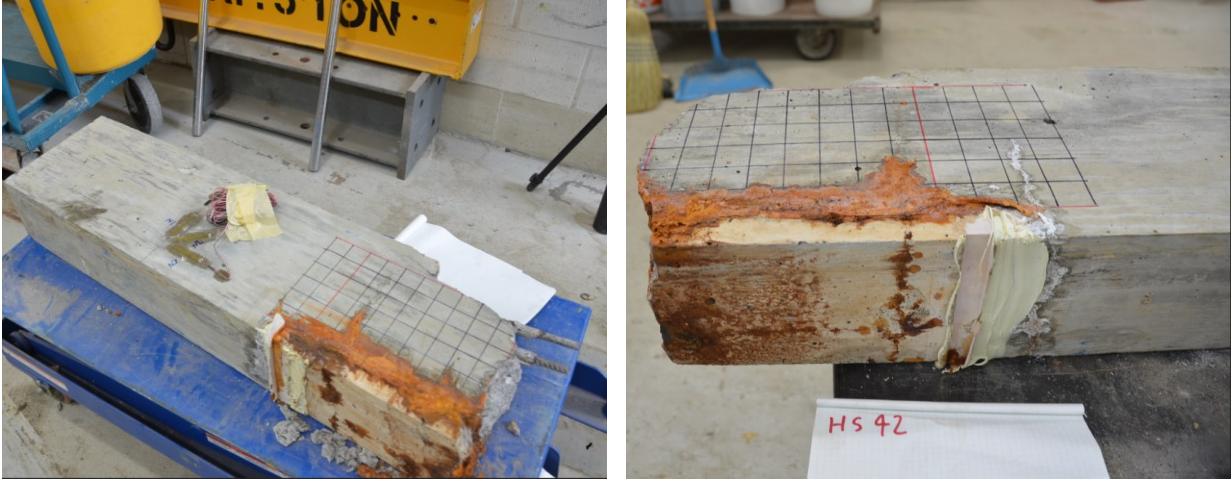
Figure A.17: Corrosion-induced damage in the cover of concrete – beam SS-2.1
