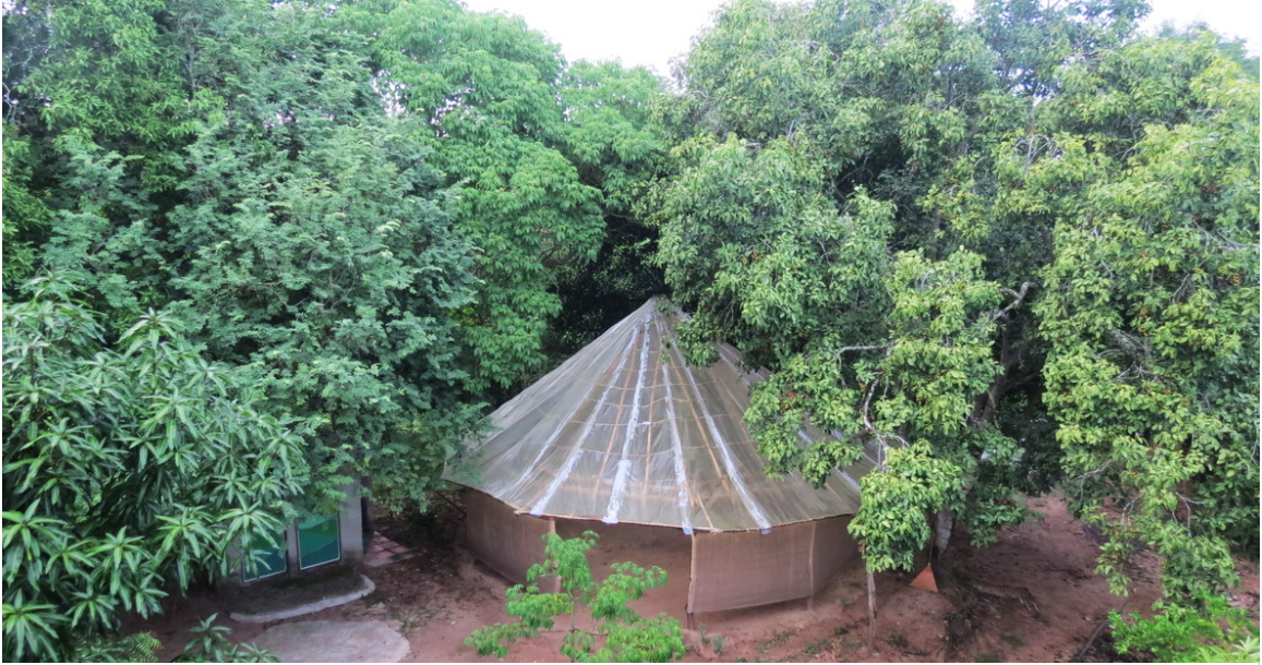
Coastal Maloca with provisional plastic roof, Casa Zindulí
