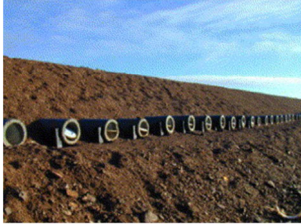
Figure 17: Duct-Ventilated fill foundation (ZHDC,2011)
