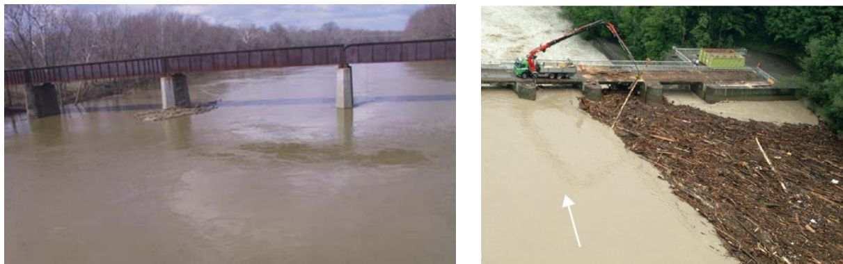
Figure 1-1(a) SRT view of the downstream railway bridge (Lyn et al. 2007) (b) large wood accumulations during the 2005 flood in Switzerland (Schalko 2018)
