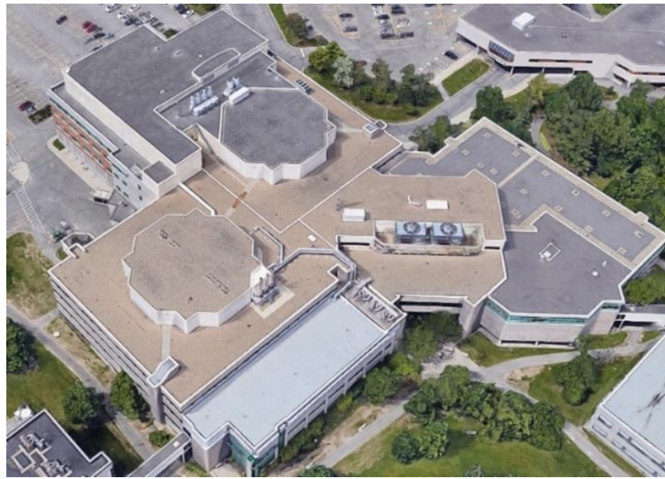
Figure 3.5 Picture of the Roger Guindon building.
