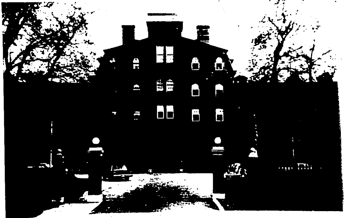
Administrative Section Viewed from King St. Source: P.A.O. RG 20, Series T-1.
