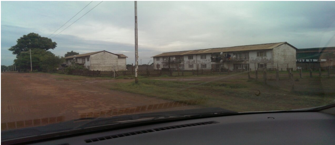
Figure 4: Dilapidated building due to environmental pollution
