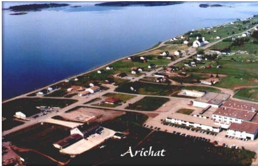
Figure 2.5: View of Low and High Roads, Arichat, Isle Madame
