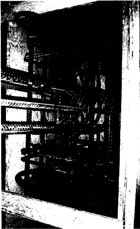
Fig. B.1 – Typical Footing Reinforcement Cage
