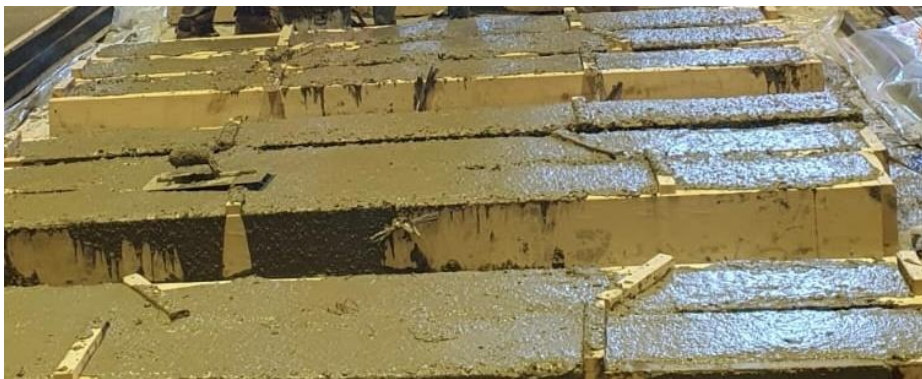
Figure 3.2 – Assembly of reinforcement cage and casting concrete.
