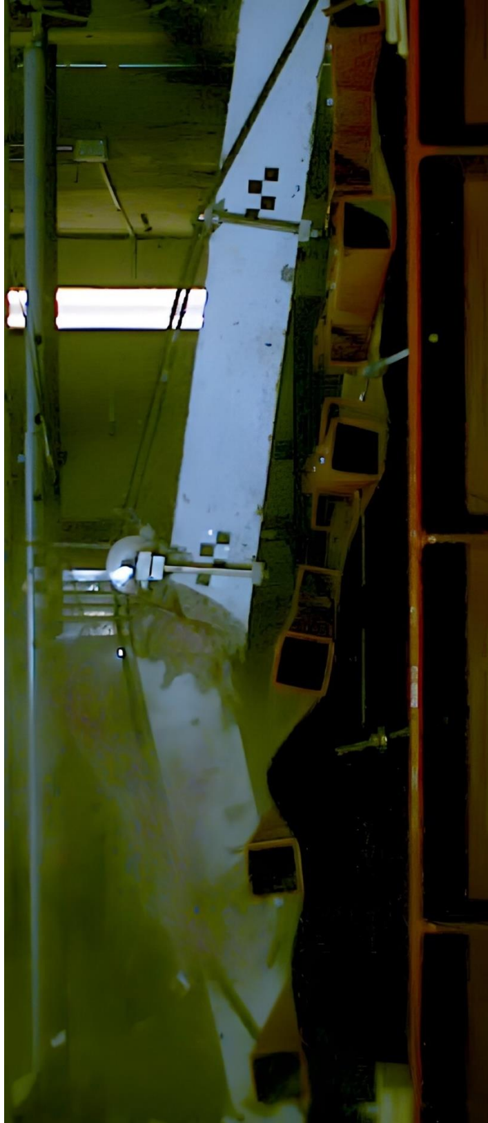
Figure 4.26 – Photos of column TH1-247e-0.10fpu-N1 after blast shot#3.
