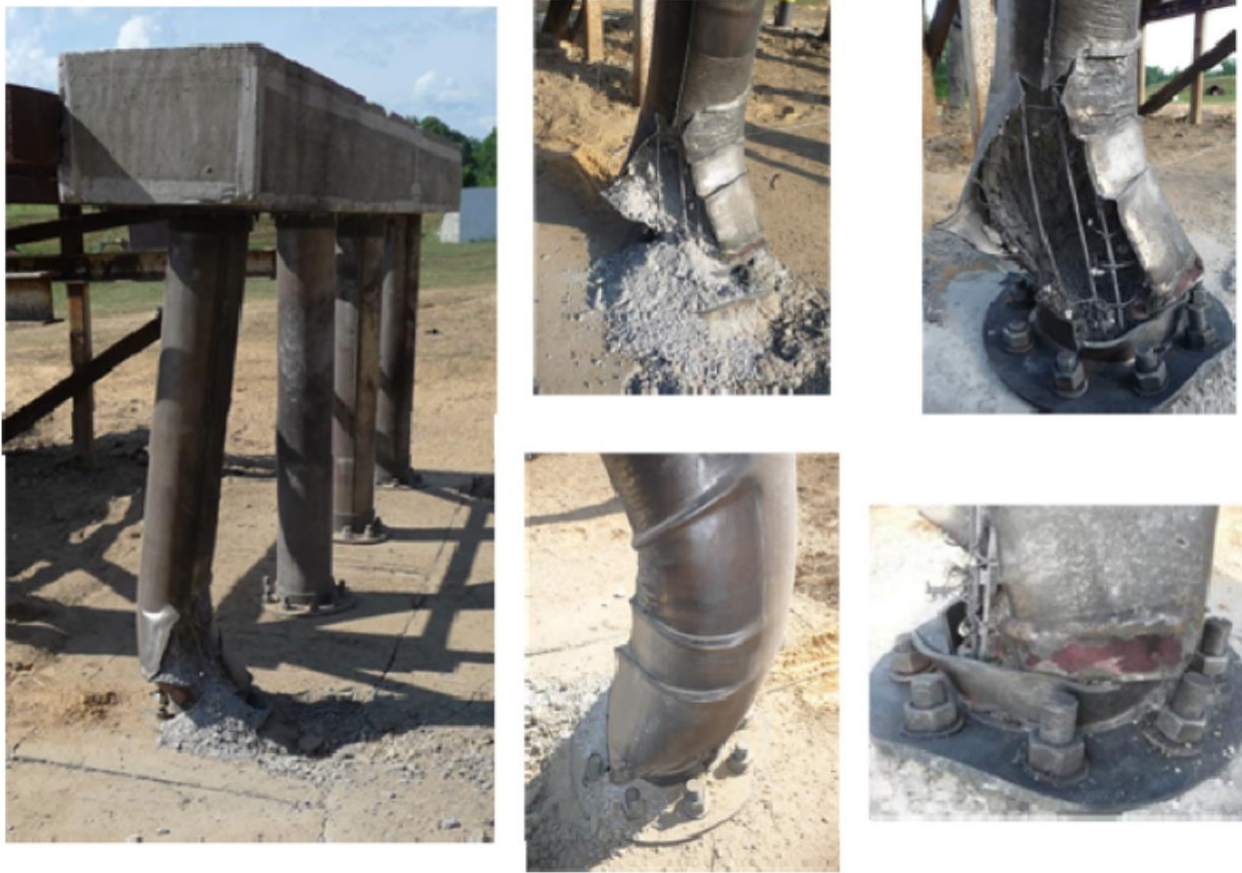
Figure 2.24 – Failure of test specimen labeled MSJC4 (global view and close up of base (source: [66])).
